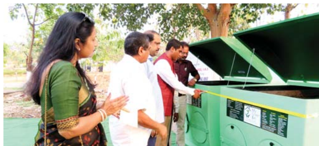
Installation of Composting Unit
